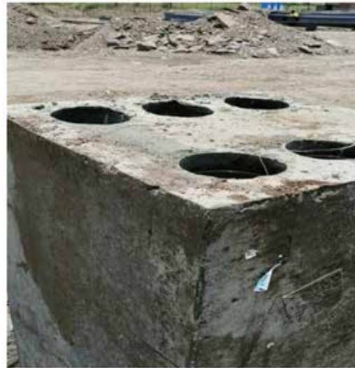
Fig. Column with Foundation Bolts after Grout
