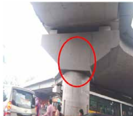
Figure 1: Pier Cap –Pier Joint of Bridge
