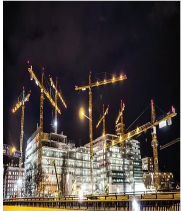
Figure 2. Working tower and Cranes
