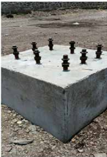
Fig. Column with Pocket Hole before Grouting
