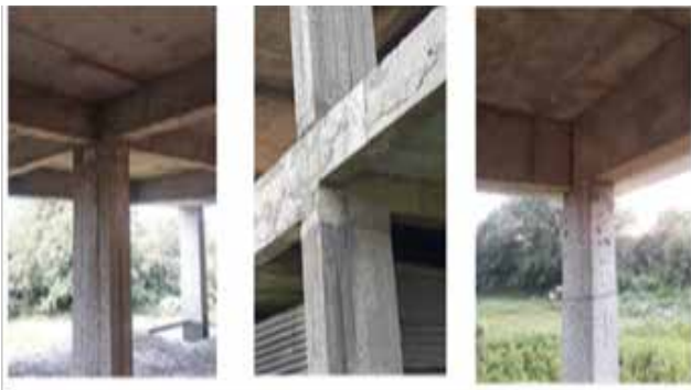
Internal Joint External Joint Corner Joint
